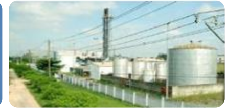
Reserved water tanks total capacity of 31,000m 3
